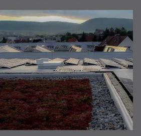
The photovoltaic plant on the green roof produces electricity, which is used for the operation of the hall as well as fed into the public grid.
